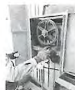
Check ชุด rapping gear EP. ( Discharge electrode / Collecting plate )/Alignment sprocket
